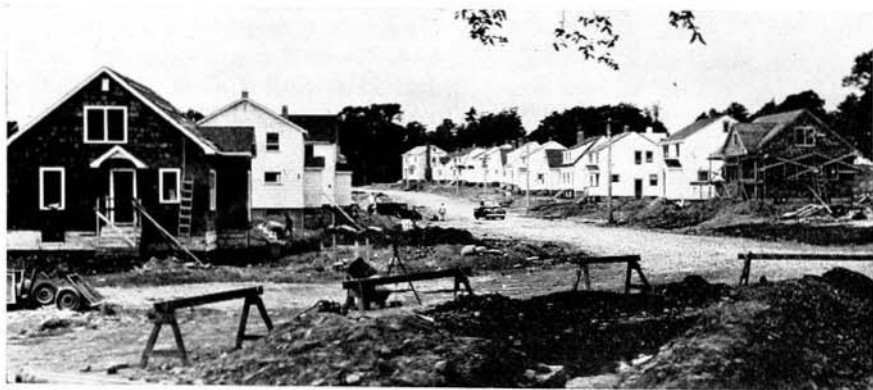
Section of Hazelhurst Sub-division, Newcastle Street
