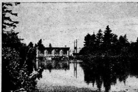
The new water pumping station at Lake Banook
