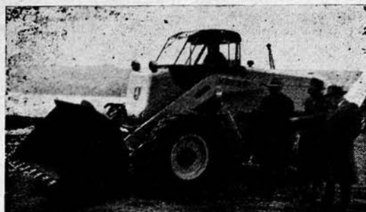
Hough loader being inspected by Town officials
