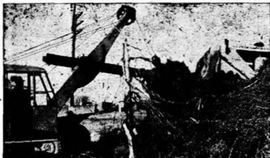
First excavation work on the Halifax-Dartmouth Bridge was started in 1951
