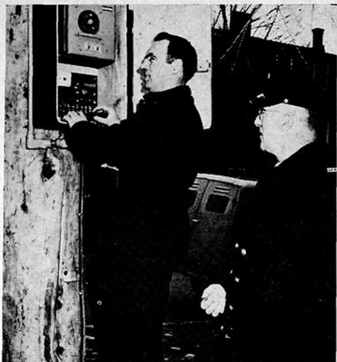
INSTALLATION OF TRAFFIC LIGHTS
