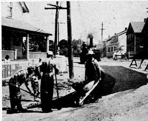
STREET REPAIR UNDERWAY
