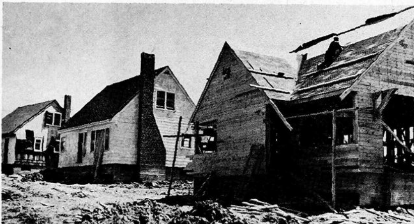
NEW HOUSES UNDER CONSTRUCTION
