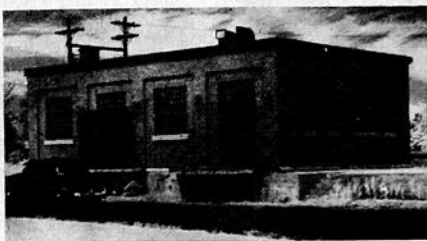
PUMP HOUSE LAKE LAMONT
