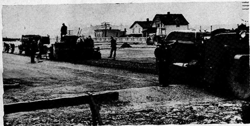
GRADING HALIFAX-DARTMOUTH BRIDGE APPROACHES
