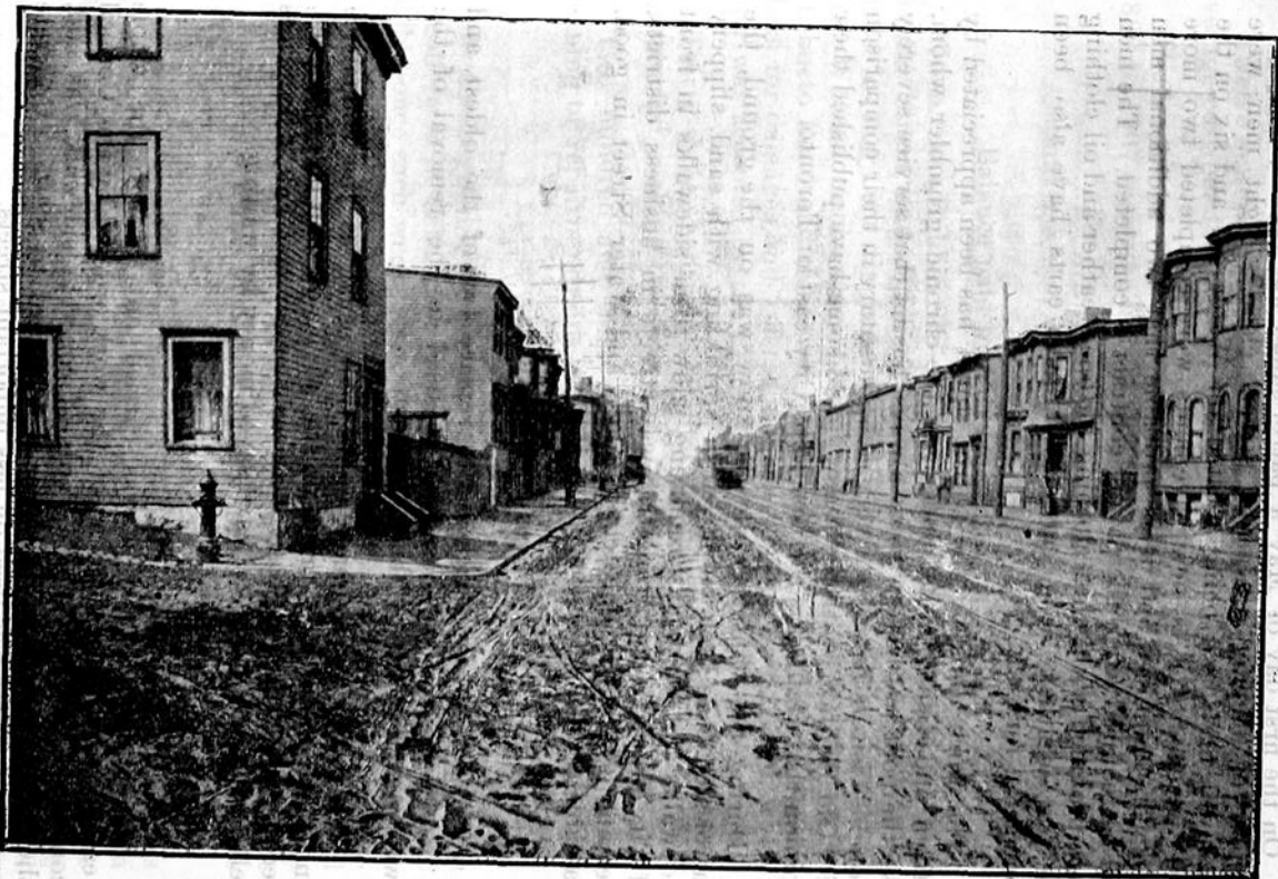
LOCKMAN STREET BEFORE PAVING.
