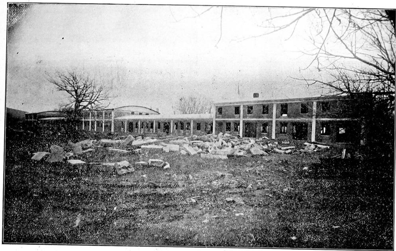
CORPORATION SHOPS AND STABLES UNDER CONSTRUCTION
