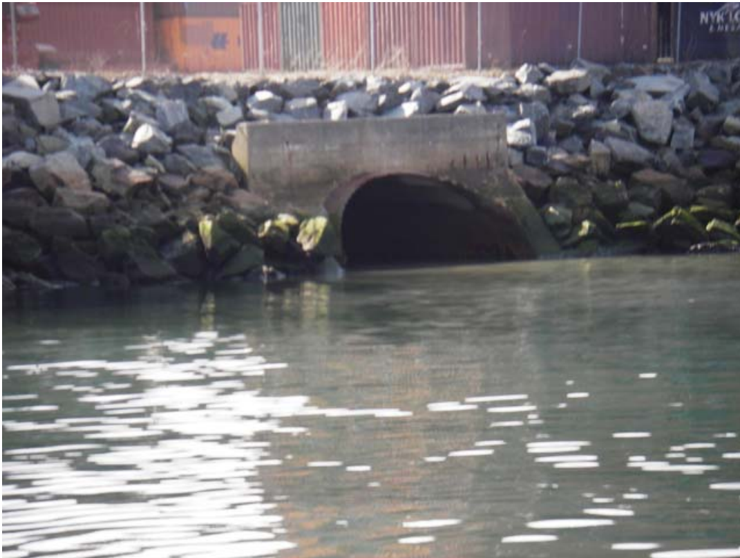
Figure 12. The Fairview Cove combined sewer overflow.
