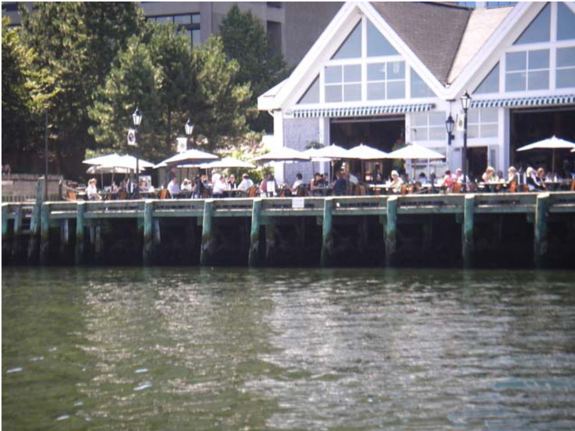
Figure 10. Approaching Harbourside Market.
