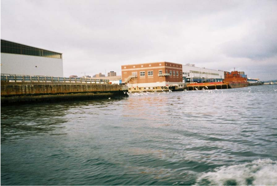
Figure 16. View looking north from inside a surface feature off Pier A.
