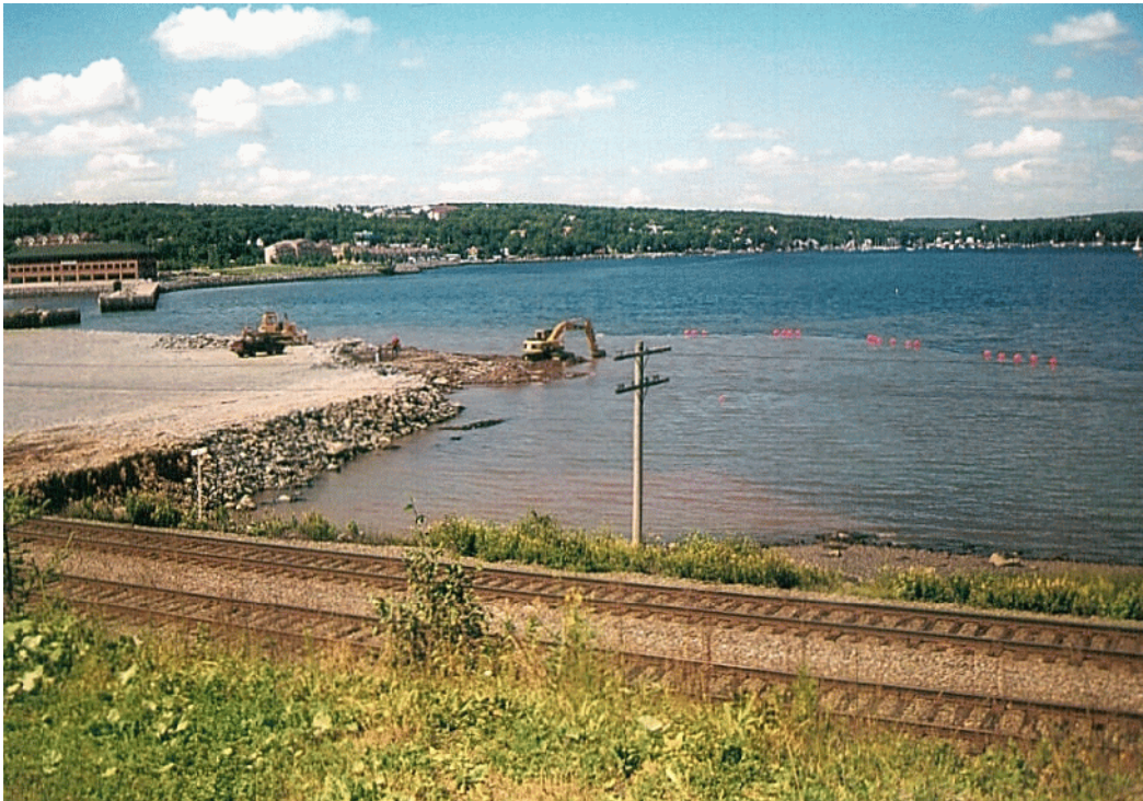
Figure 6: Phase two Bedford Basin infilling operation. Acidic rock is deposited below the low water mark and covered with standard rock fill. Silk curtains suspended from the red buoys minimize the migration of silt from the area.
