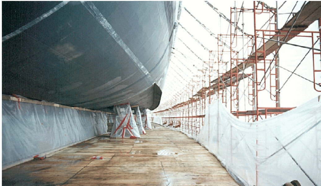
Figure 3: Close-up view inside canopy showing sealed plywood decking on synchrolift plus sheathing to prevent dust emissions and paint overspray losses. All wash water and associated debris is collected for treatment or disposal. This canopy reduces weather downtime and offers better climate control for paint application.
