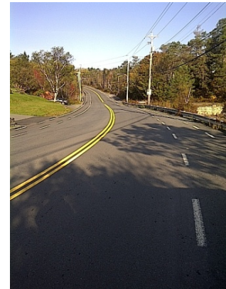
Purcell's Cove Road – Area 1
