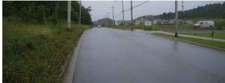
Photo 1 - Looking south on Walker Avenue towards the Self Storage / Wheatons' driveway from the west site driveway south of Sackville Transit Terminal.
