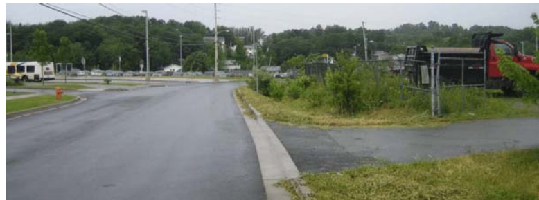
Photo 2 - Looking north towards Sackville Transit Terminal and Old Sackville Road from the west site driveway near Wheatons' driveway. Sight distance to the north can be improved by removal of bushes on the inside of the curve at the top of the photo.
