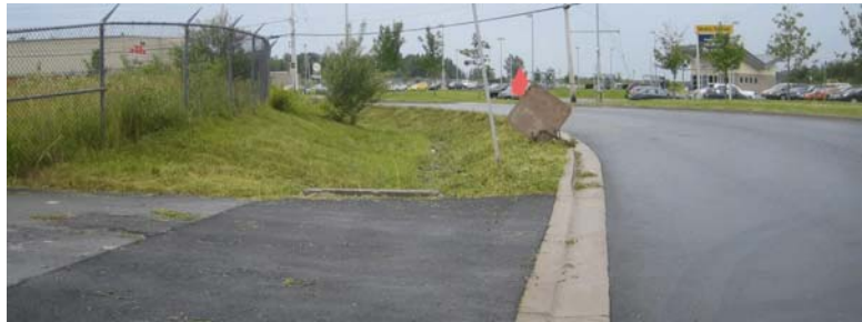
Photo 3 - Looking west on Walker Avenue towards Sackville Transit Terminal at the north site driveway to the underground parking level. Sight distance to the west can be improved by removal of bushes on the inside of the curve.
