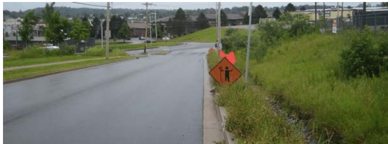
Photo 4 - Looking east on Walker Avenue towards Old Sackville Road from the north site driveway to the underground parking level.
