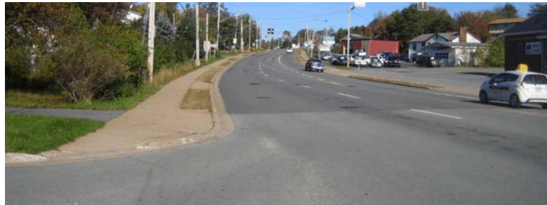
Photo 1 - Looking west on Sackville Drive towards the proposed new driveway from the existing Kent site driveway. Note the beginning of the eastbound left turn lane to the right of the photo and the westbound left turn lane at the top of the photo.
