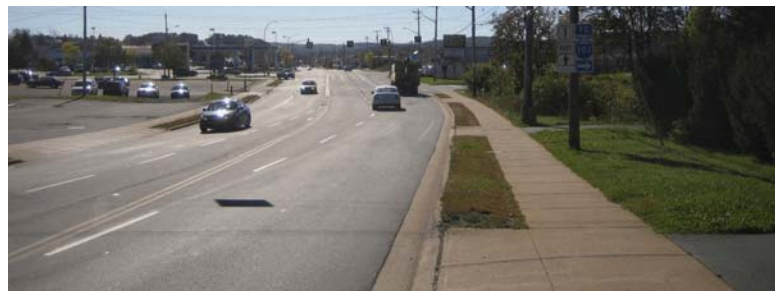
Photo 4 - Looking east on Sackville Drive towards the existing Kent site driveway and Beaver Bank Road from the proposed new site driveway. The transition from eastbound to westbound left turn lanes is visible in the lower left of the photo.
