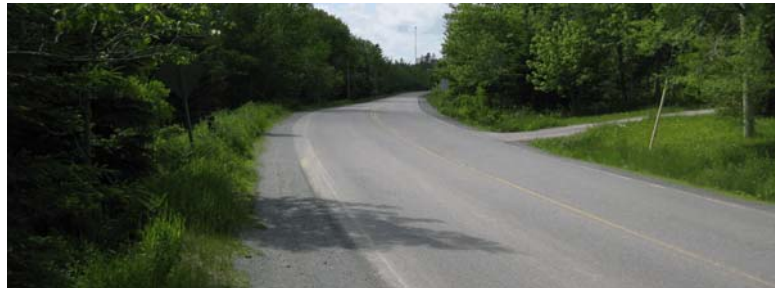
Photo 1 - Looking west on Sackville Drive from near the east Abandoned Road intersection.
