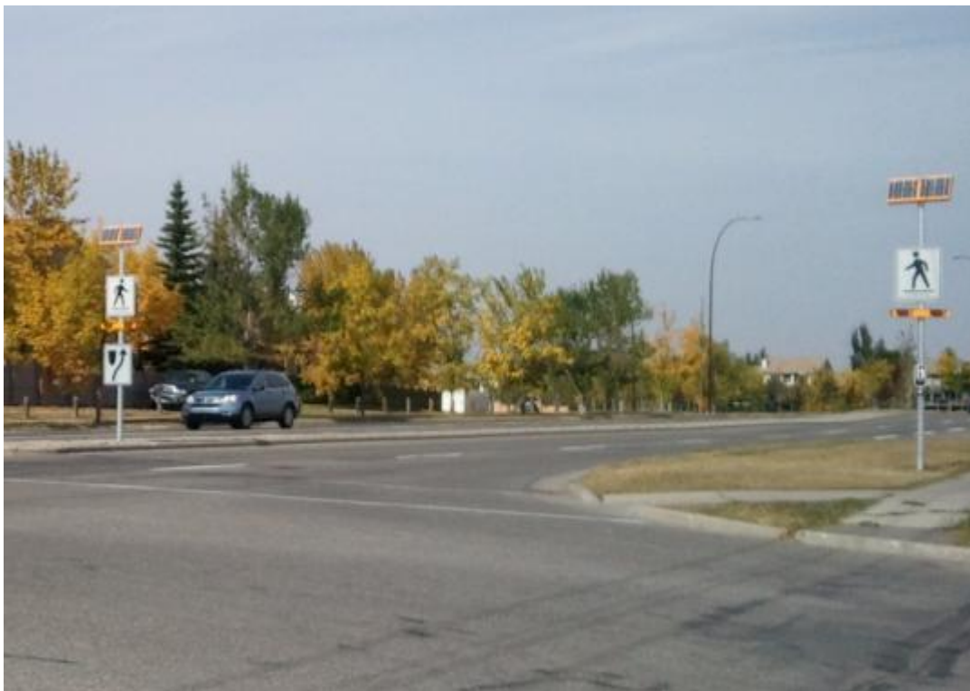
Crosswalk Upgraded with RRFB in Calgary
