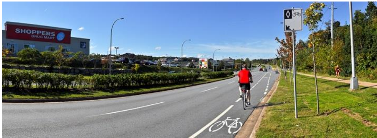
Dunbrack Street Bicycle Lane
