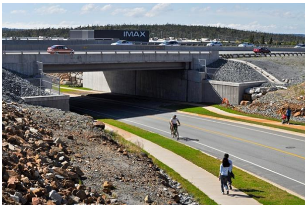
Washmill Lake Road Underpass
