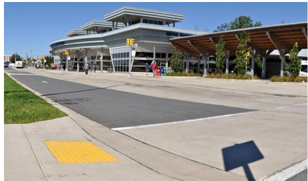
Tactile Markings at the Bridge Terminal
