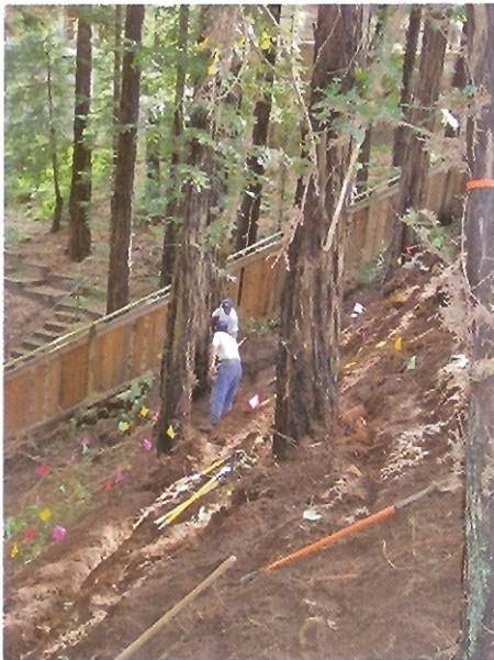
A steep slope installation in California — 65% slope.
