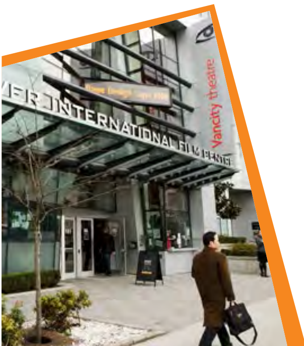
Vancouver International Film Center • Vancouver, BC Developers of the Brava tower paid $5.0 towards the construction and operating costs the VIFC to increase FAR from 5.0 to 8.08.
