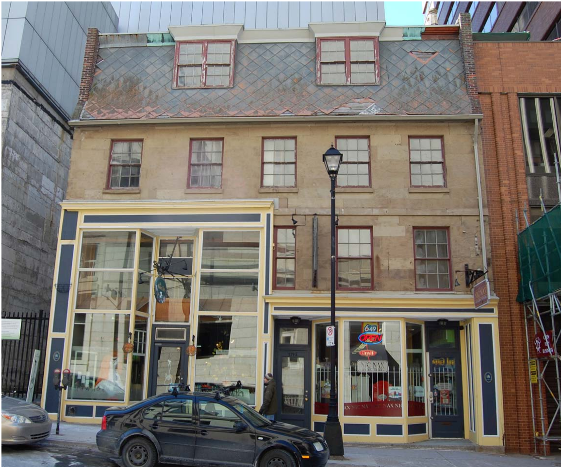
Macara-Barnstead Building, Granville Street façade, 2011
