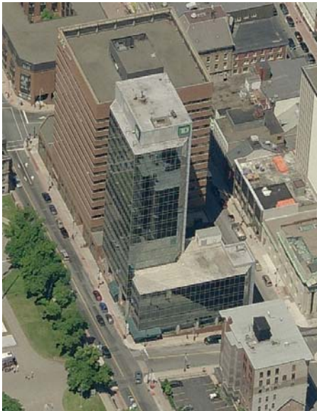
Aerial view from southwest
