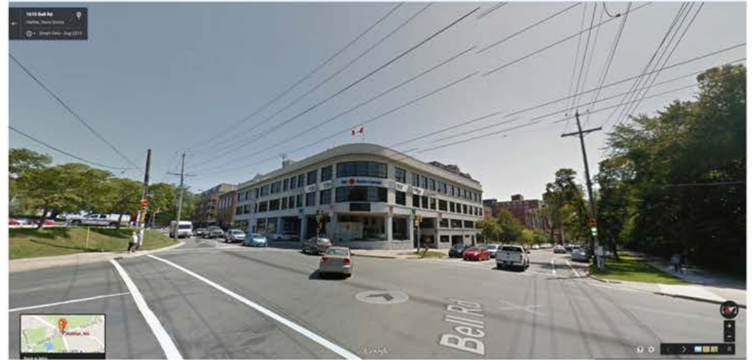
VIEW FROM INTERSECTION
