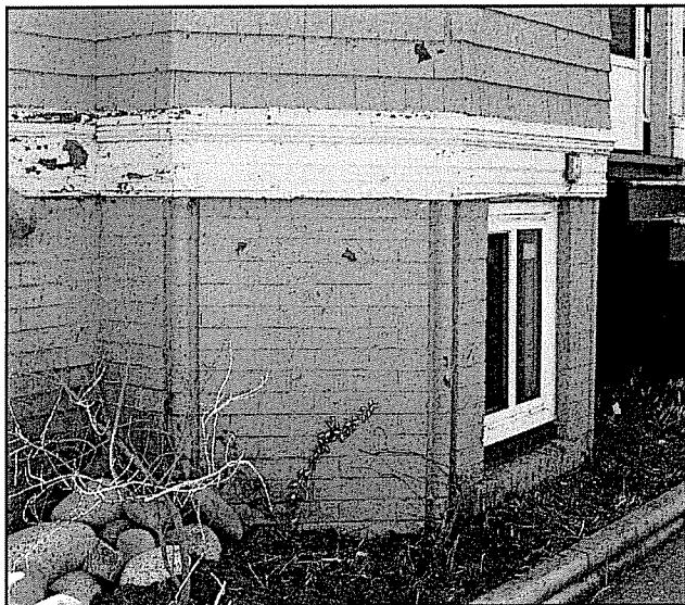
Foundation, 5516 North Street.
