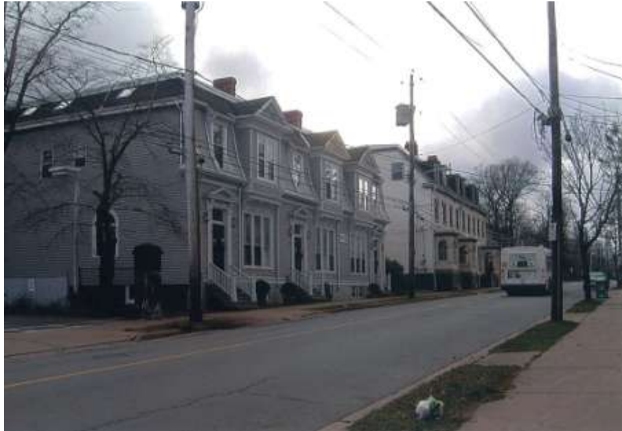
Front and east elevations. Susan Little 2012.
