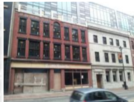
1652-62 Barrington Street 8,821 sq ft total lot area on rising grade
