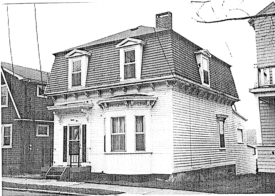
Photo 3: Photograph from Heritage Property File, c. 1983.
