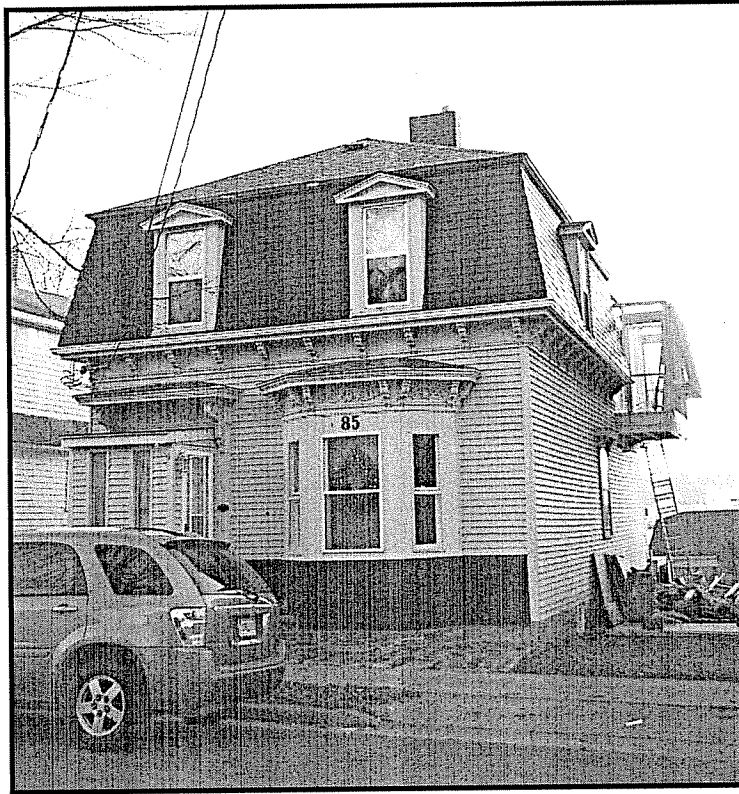
Photo 1: 85 Fairbanks – Front and west elevation: the cantilevered addition is visible.
