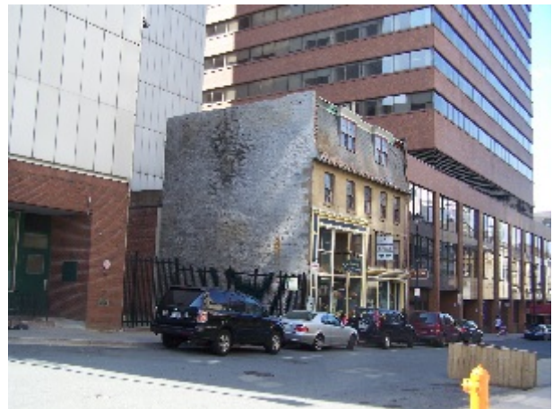
Macara-Barnstead building 2011. Whitewashed side wall highlights sandstone corner quoins.
