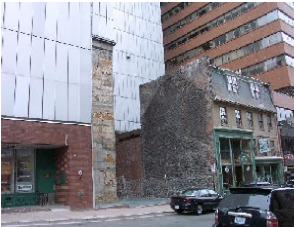
Original truncated gable-roofed form of Macara-Barnstead Building revealed in stone side-wall after demolition of Kelly Building in 2006. The 1880s rear addition can also be seen. Original chimney pots can also be seen above the roof line on the north side (there are fireplaces in each of the upper floor rooms).
