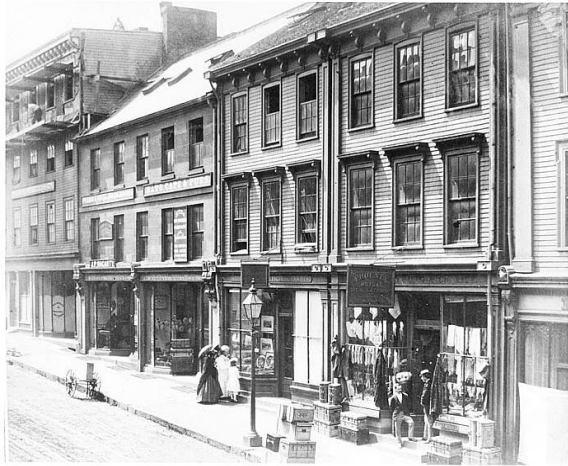
Earliest photo of Macara-Barnstead building, from Roger's Photographic Advertising Album, 1871. Kelly building is on the extreme left. Macara-Barnstead second from left, showing storefronts renovated in 1860s and occupied by Hagarty's Musical Instruments on the left and Everette's Hats & Furs on the right.
