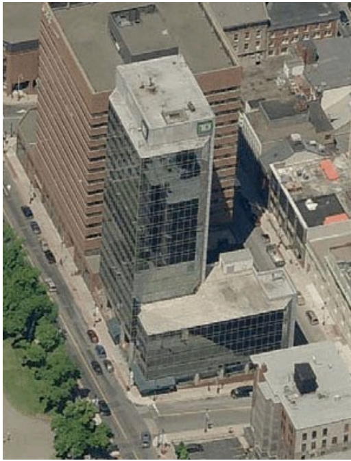
Existing TD Centre Aerial View Front
