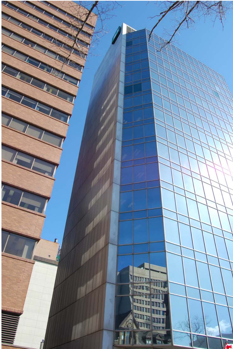
View of northwest corner of tower showing blank wall facing CIBC building
