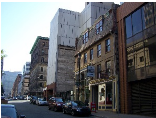
Macara-Barnstead building is slightly "proud" of adjacent CIBC building, revealing sandstone corner quoins.
