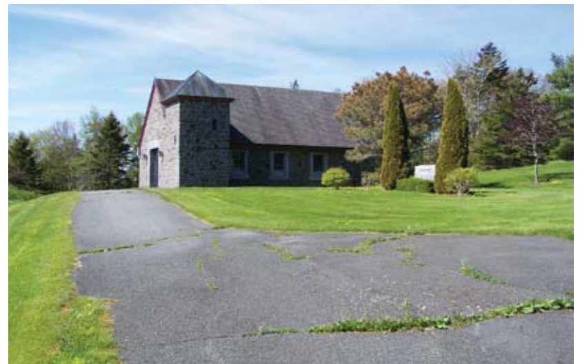
2014 Photo of Santa Maria del Pilar Chapel
