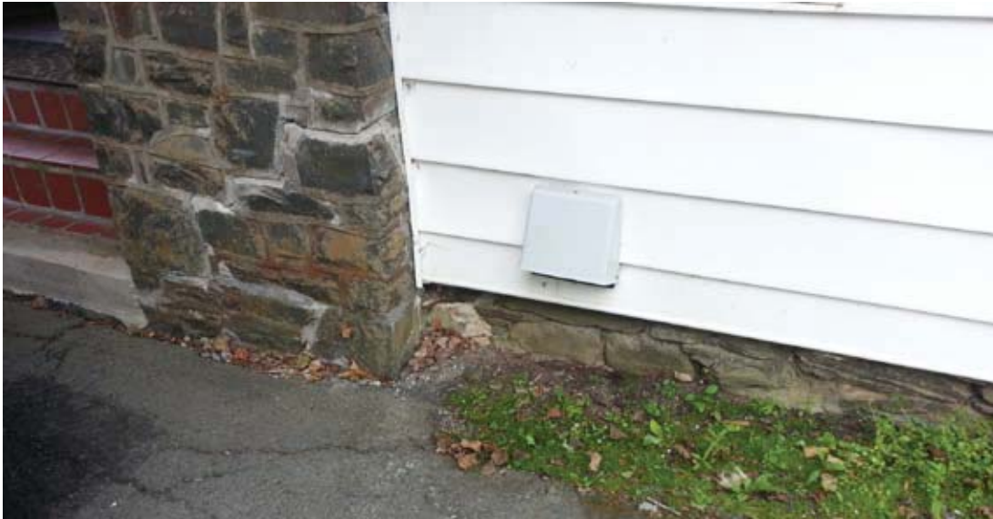
2014 View showing stone foundation of main house adjacent verandah
