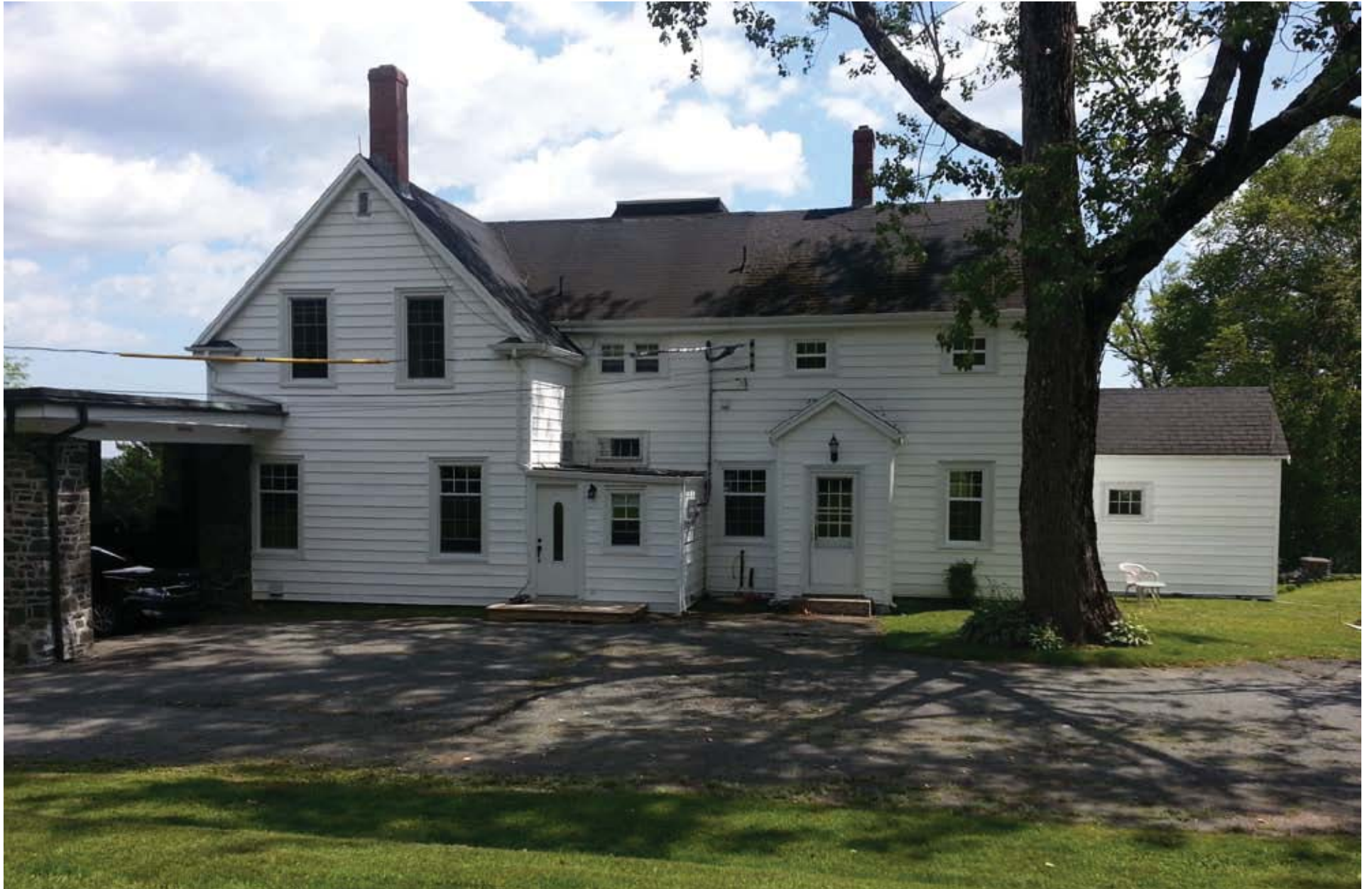
2014 View of Lindwood House - View from driveway (North side)
