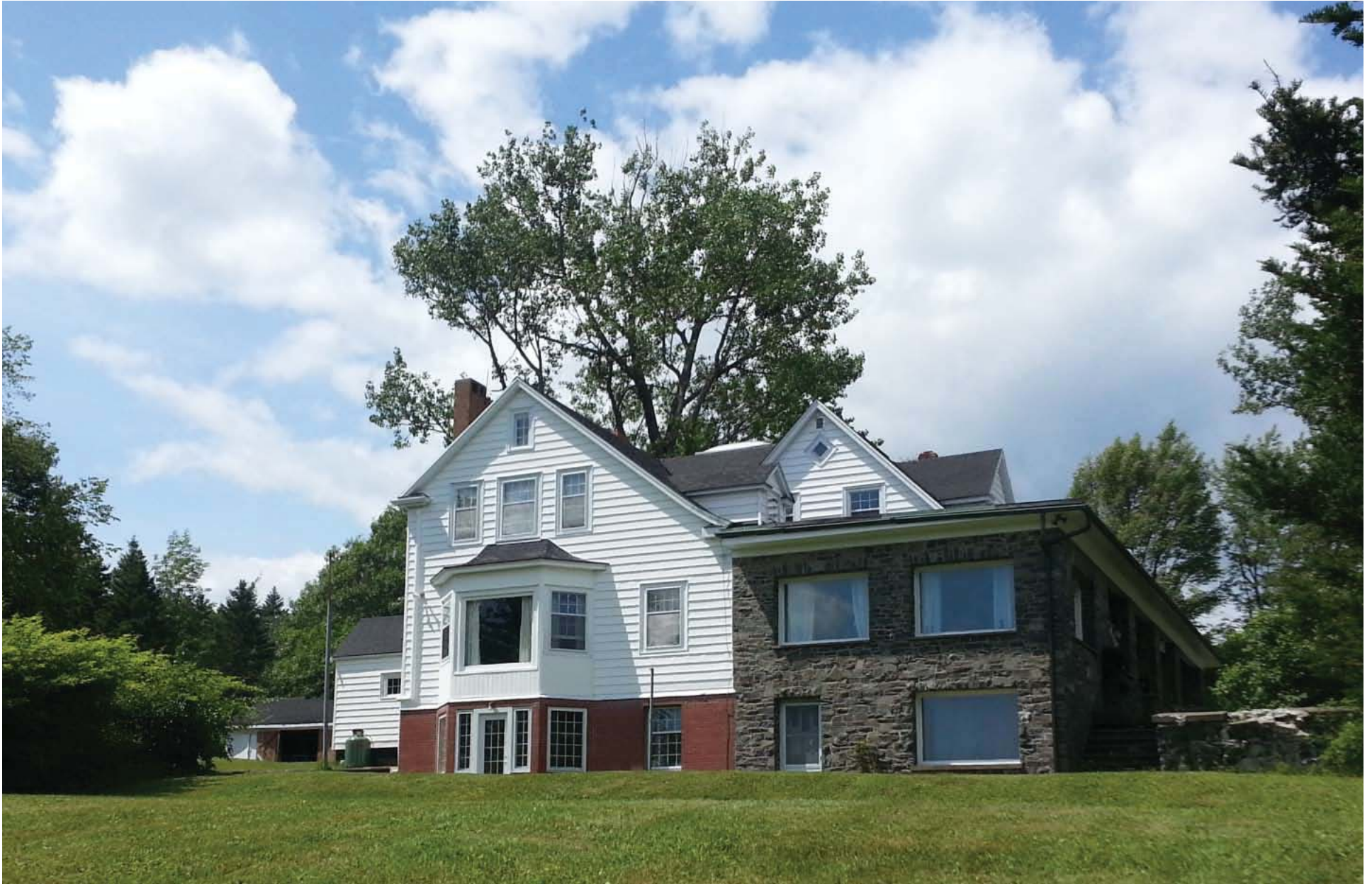
2014 View of Lindwood House with garage in background - View from lawn (South side)
