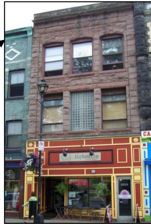
1725 Barrington Street Cabot Building
