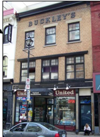
1667 Barrington Street Buckley's Building
