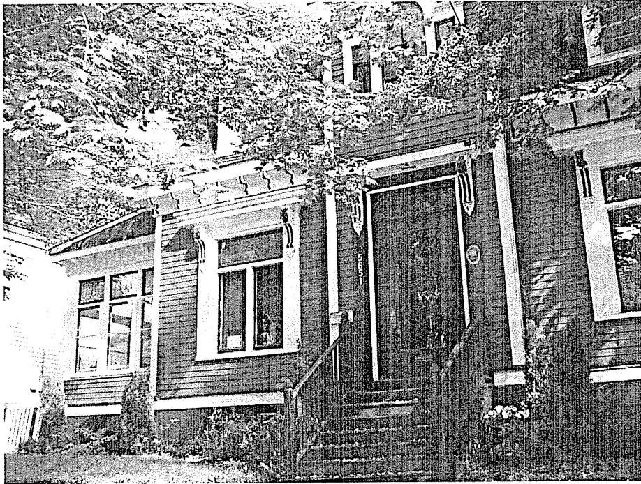
Figure 1: Front elevation of 5651 Inglis St, Halifax.
