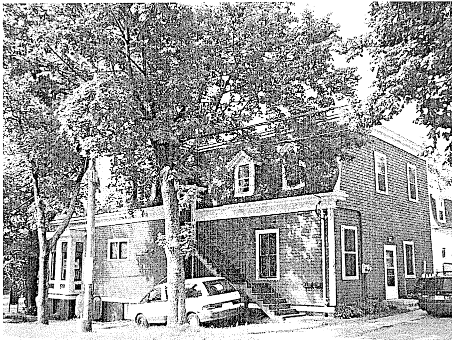
Figure 4: Side and rear elevation from Lucknow Street.
