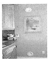
Installation is very simple. By cutting an intake and exhaust diffuser hole, the panels are typically mounted on the south facing wall of a building (you can see the inside diffusers on the third picture above). A solar powered fan draws air from the house into the panel, it is heated by the panel and then exhausted back into the home.
