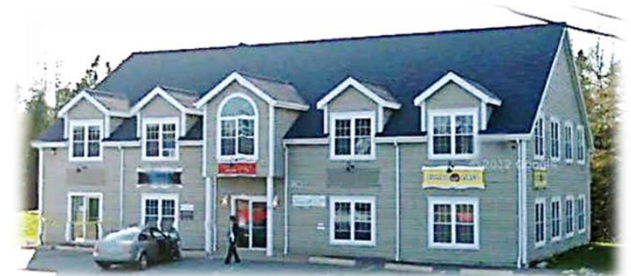
Photo Credit: Google Streetview, 2013
