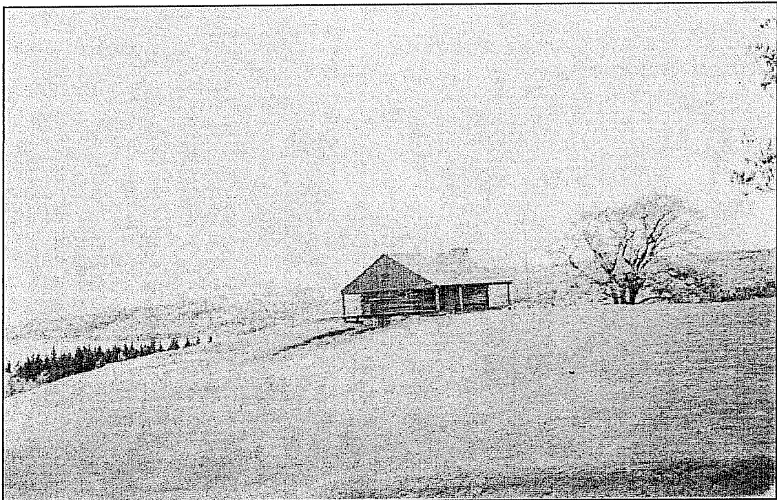
Figure 2: Photograph of the Bedford Golf Course Clubhouse, date unknown.
