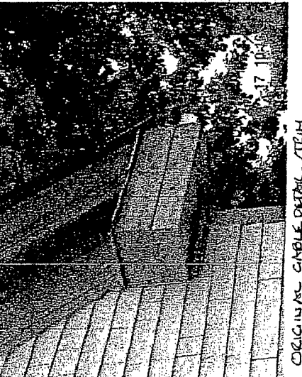
INAPPROPRIATE TRIM - RESULT OF REPAIR
