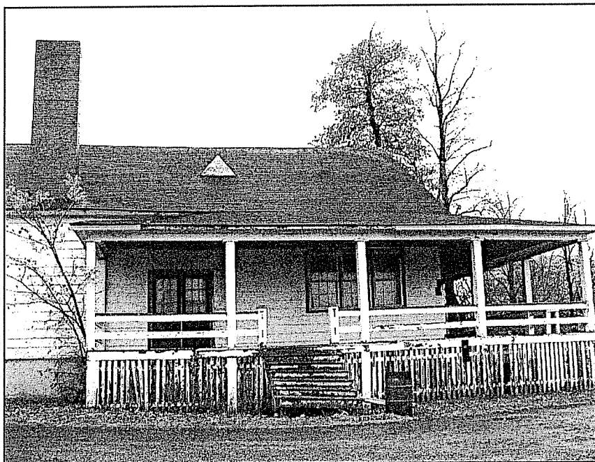
North facing elevation of the Dry Canteen.
