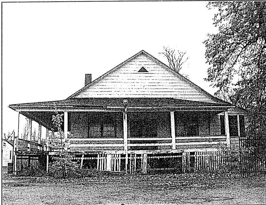
West facing elevation of the Dry Canteen.
