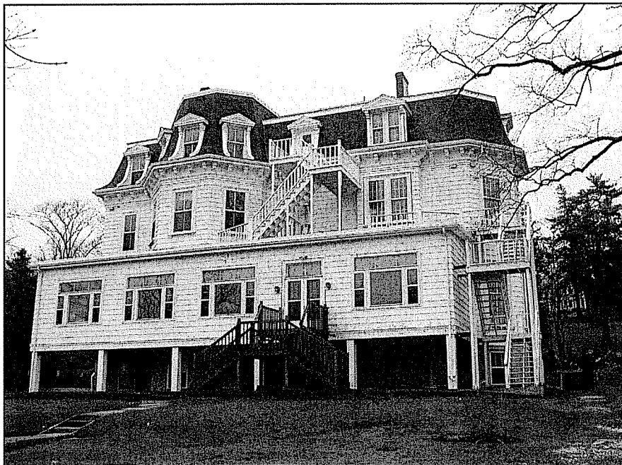
Rear, or waterside, elevation of 1390 Thornvale Avenue.
