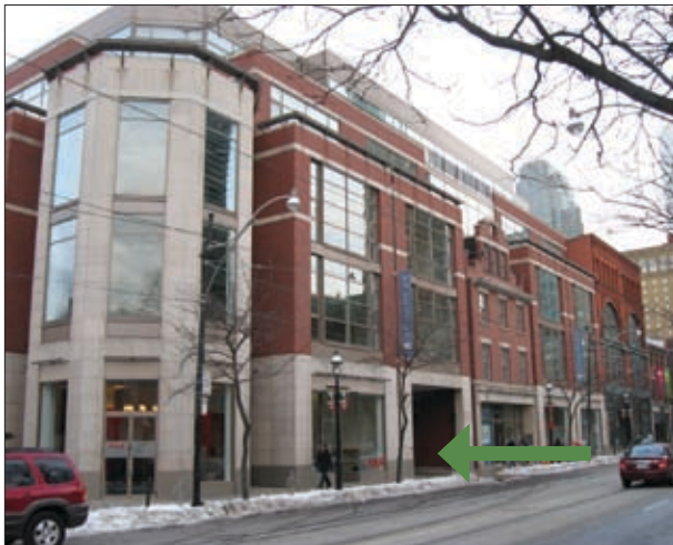
Service vehicle access is through an access portal integrated with building façade. The width of the frontage it occupies is minimal.
