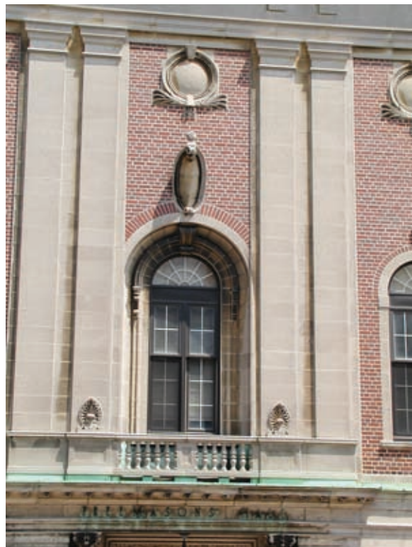
Brick cladding with sandstone pilasters and window surrounds
