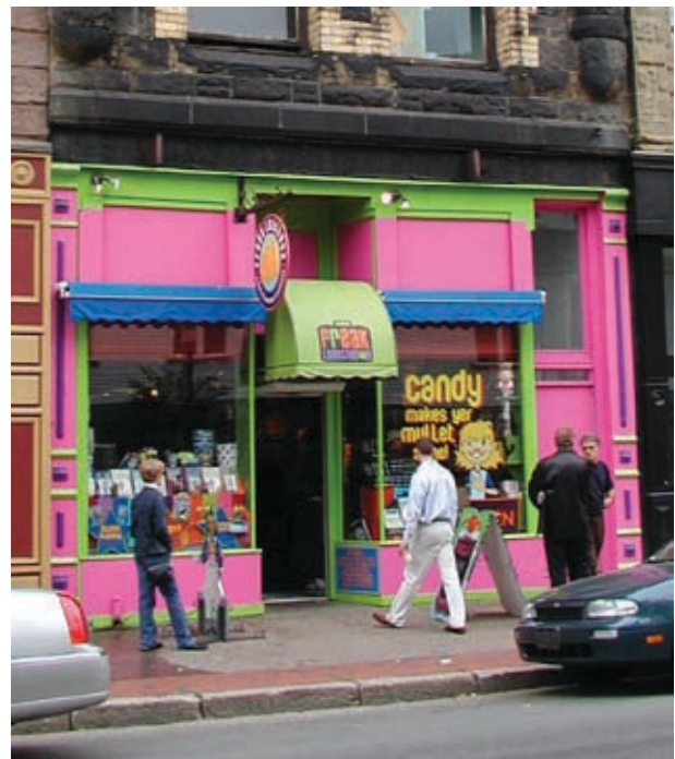
Here, an unsympathetic paint scheme has created a vivid contrast with exterior masonry on the upper facade and obscured architectural detail within the storefront
