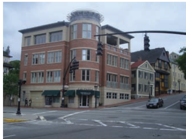
Material variety used to articulate the building: stone base, brick facade and a variety of details to articulate the base, middle and top. Materials wrap visible facades.
