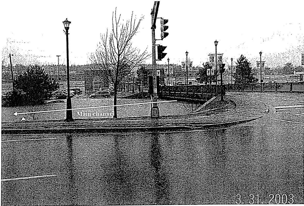
(Downstream Side of Towers Bridge)
