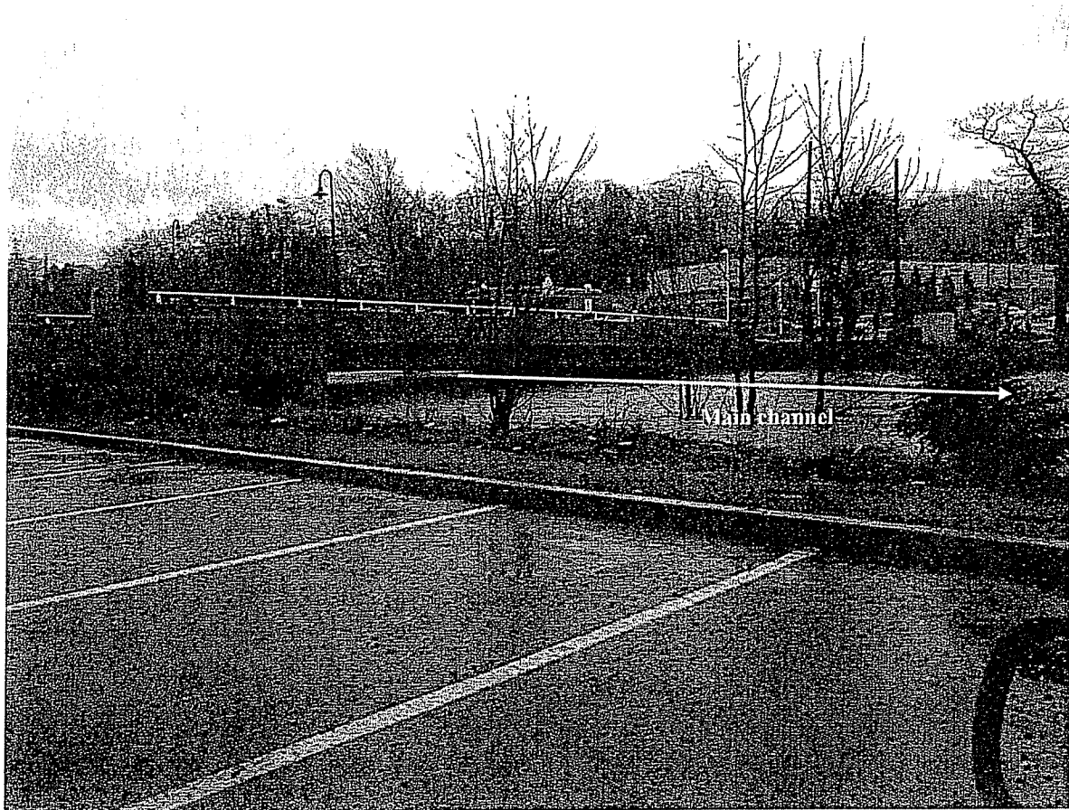
(Downstream Side of 2002 Bridge)
