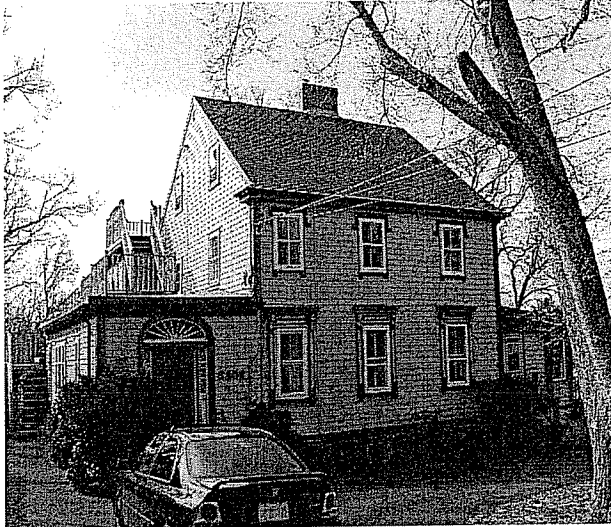
View from Coburg Road
