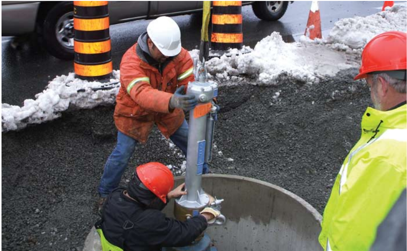
Lowering the PipeDriver™ into the launch chamber to inspect the 30 inch pre-stressed concrete pressure pipe on Hammonds Plains Road
