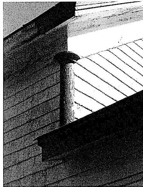
Detail: corner boards with the appearance of engaged columns.
