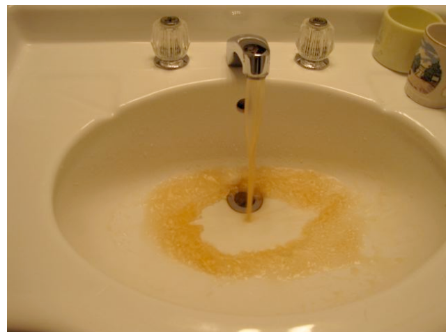
Figure 7 - Discoloured water, after running a minute, Sept.10/09
