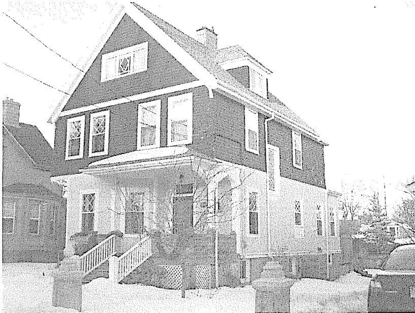
Front and South side
