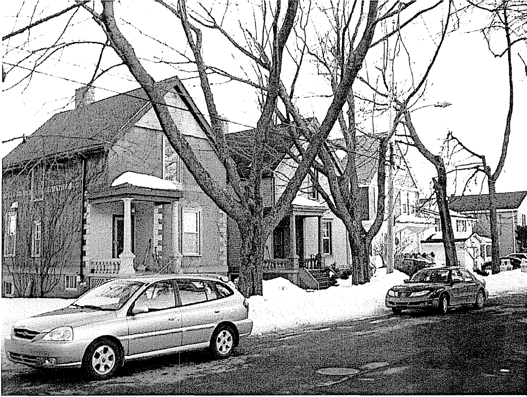
Two adjacent houses (1155 and 1149 Cartaret Street) also built by George B. Low
