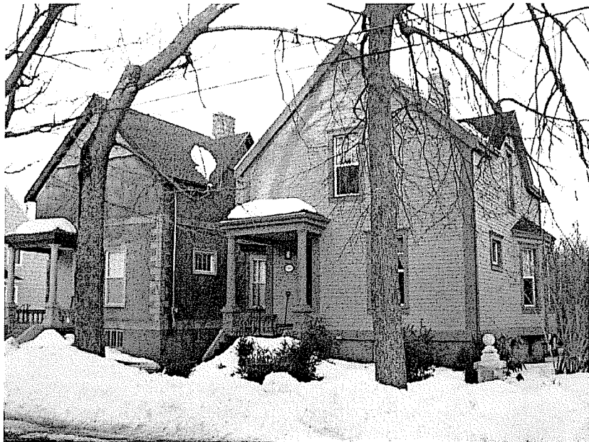
1155 Cartaret has original concrete exterior; 1149 Cartaret has been re-clad with wooden shingles
