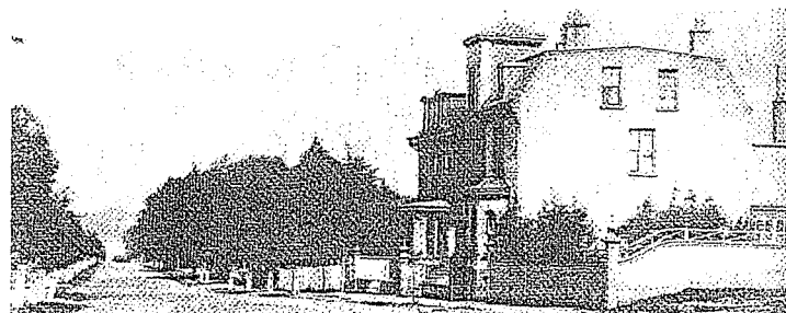
Uniacke-Sawyer house. (Courtesy of NSARM)
