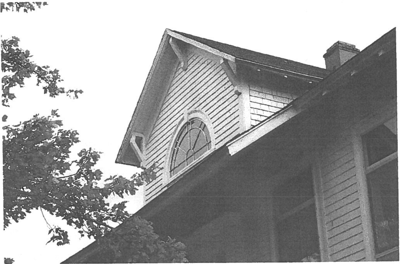
Front dormer showing knee braces (photo by Colette Bishop-Greene, 2012).
