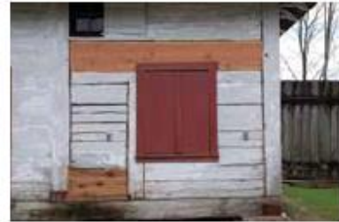
A condition assessment of the exterior walls and frame of this Storehouse at Fort Langley, BC found extensive deterioration of some timbers, which required replacement in kind. The dimensions, hewn finish and species of wood used in the repairs matched those replaced. The photograph shows part of one storehouse wall after the repairs were completed, but before the new timbers were whitewashed.
