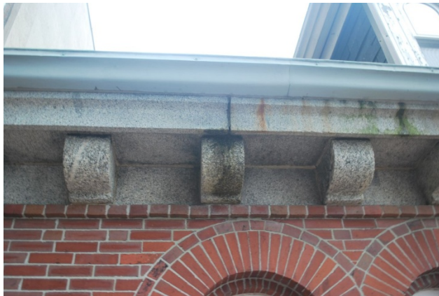
Fig 13. Showing ferric staining, biogrowth and other general forms of surface dirt on the surface of the gutter level granite. Each can be removed with relative ease.
