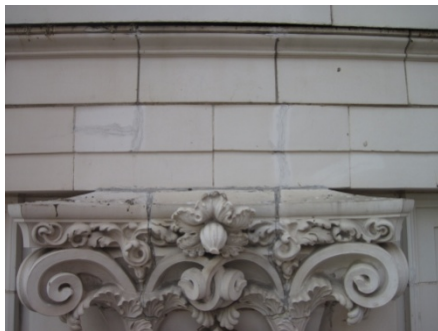
Fig. 27. Typical twin vertical cracks or fissures observed above Coninthian Capitals. Further consideration of this issue by a Conservation Engineer is recommended.
