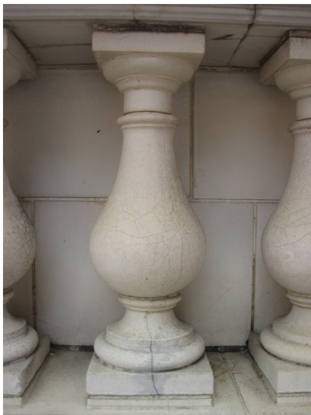
Fig. 16. Showing typical hairline crazing of terracotta surface.
