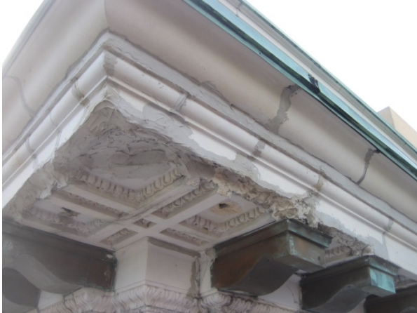
Fig. 19. Polyester resin, essentially auto body repair material used to adhere and patch severely deteriorated and dangerous overhanging terracotta.
