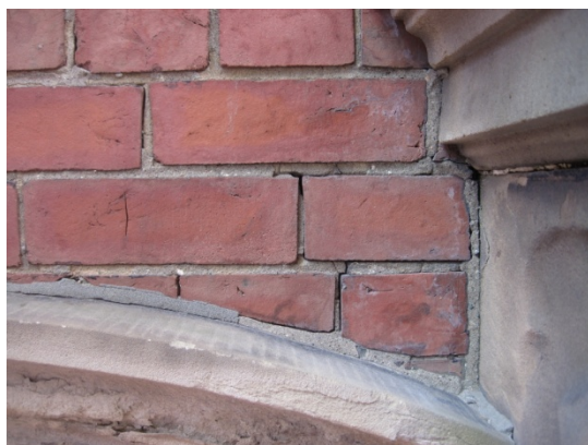
Fig. 31. Showing typical good condition of brick, but poor condition of the joint mortar. Shallow and superficial repointing of the past can be seen here.
