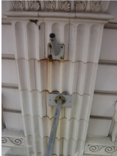
Fig. 26. Ferric staining from fasteners used to anchor fixings.
