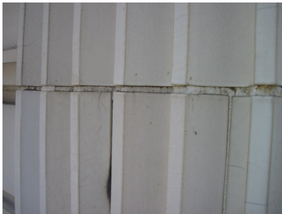
Fig. 24. Original mortar. Showing weathering, cracking, attrition.
