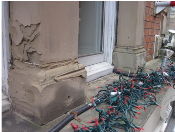
Fig. 33. Major deterioration of decorative surface, despite being properly bedded in natural orientation.
