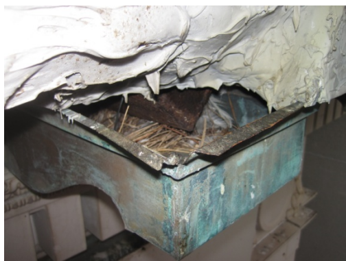
Fig. 18 showing the corroded iron anchor support of cornice.
