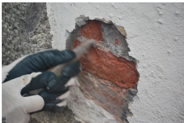
Fig. 36. Small opening suggest, spalled brick covered with a hard render layer (dark colour) and topped with a white polymer coating. Note the adhesions of the render to the original brick face, which would be near impossible to remove if there was any wish to remove render to original brick face.
