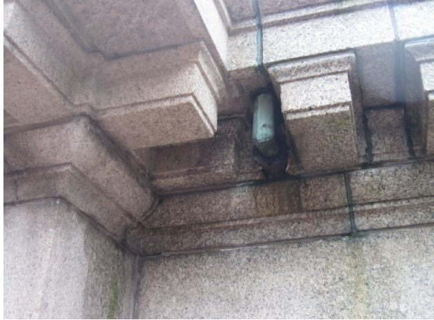
Fig. 4. Down pipe dysfunction. Masonry spreading as witnessed by joint movement. At very left, fracture of moulded stone a result of exerted lateral forces.
