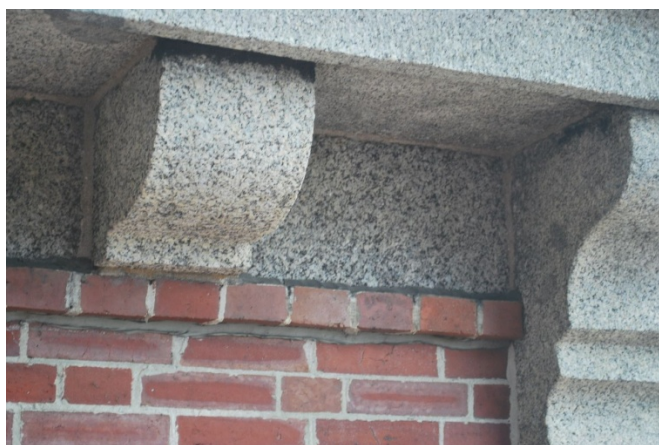
Fig. 12. Hard dense repointing mortar located at the upper granite and first course of brick. This suggests needed maintenance work to keep joints sealed in. However, it may mean another issue of leakage at roof and gutter is present.
