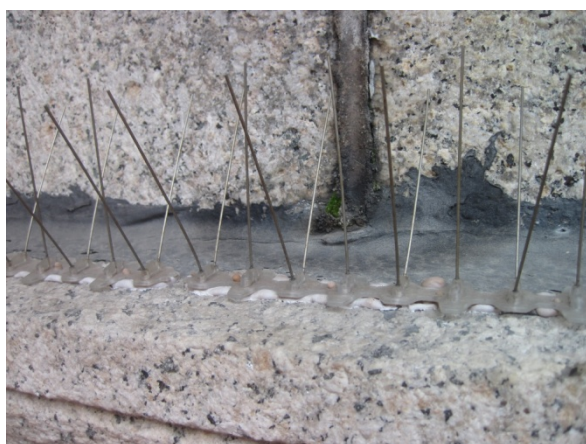
Fig. 6. Note the growth of moss in the saturated mortar joint. Also, typical bird deterrent and related tar adhesive to typical at top of ledges.
