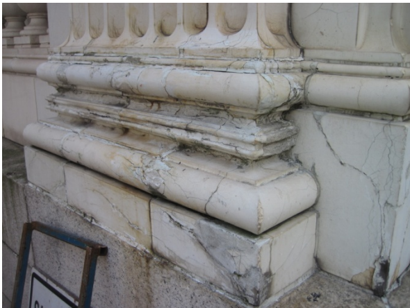
Fig. 20. Showing excessive use of polyester resin repairs. The condition of the terracotta is far beyond repair.
