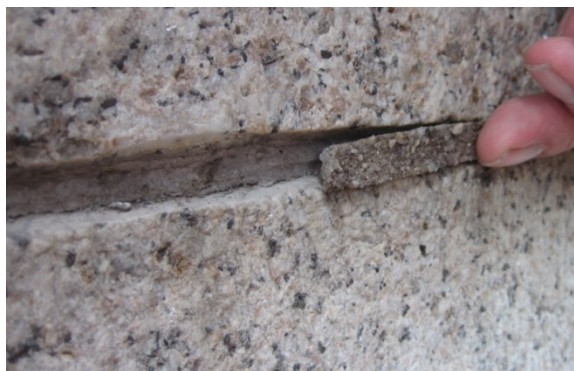
Fig 2. Note shallow repointing, lack of bond, widening of joints
