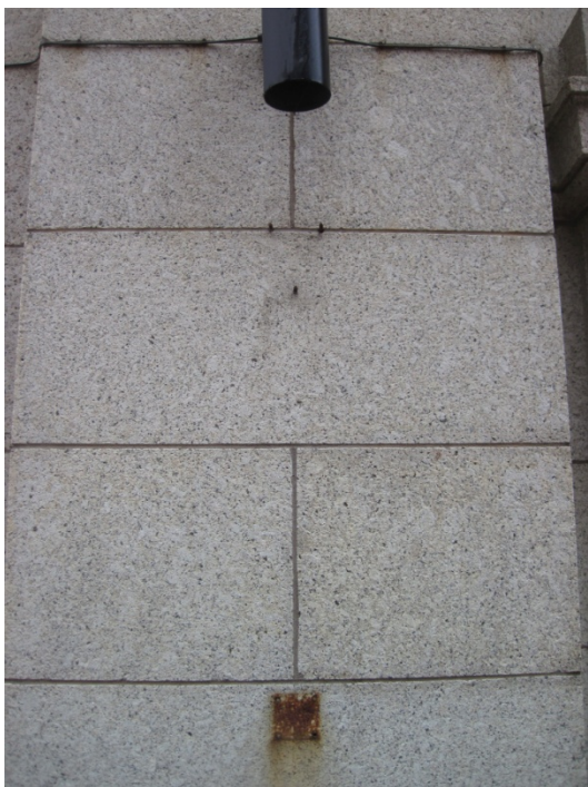
Fig. 5. Ferric staining marking otherwise clean wall.
