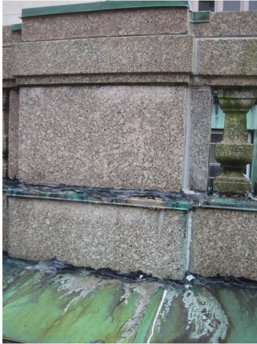
Fig.2. Precipitate salts from water infiltration. Caulking and tar in efforts to stem falling water through the masonry.
