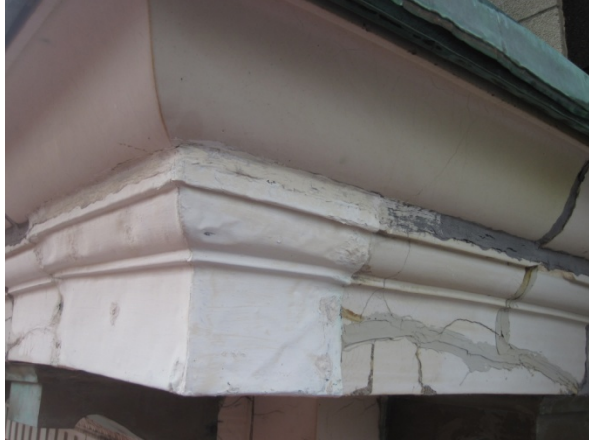
Fig. 21. Showing sheet metal tin to repair, conceal, and replace
