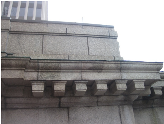
Fig. 3. Substantial lateral movement of the parapet wall.
