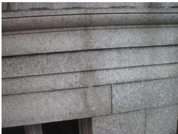
Fig. 8. Difficult to see, but vertical crack at window upward.
