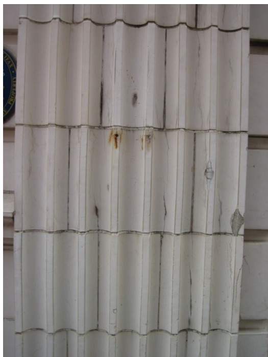
Fig. 23. Fissures and spalls, some previously filled with mismatching materials and colours, can be made good by cosmetic conservation repairs.
