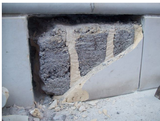
Fig. 17. Showing grout (and brick) filled core of terracotta unit.
