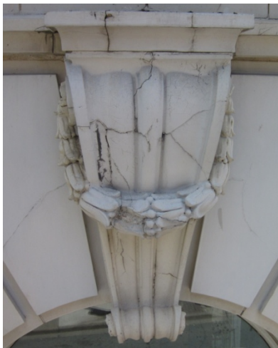
Fig. 29. Decorative key stones are all in good preservation except this one at the north elevation, west side. Major fracturing will mean replacement is necessary.
