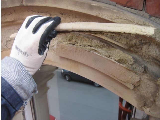
Fig. 32. Major deterioration and loss of decorative moulded window stones. Extensive replacement is necessary.
