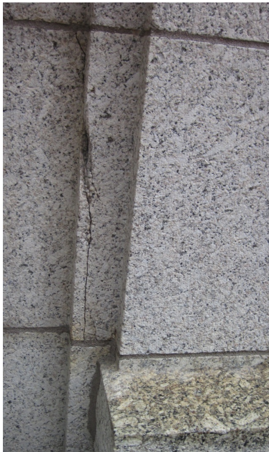
Fig. 9. Fractured stone due to isolated loaded of stone along vulnerable detailing.
