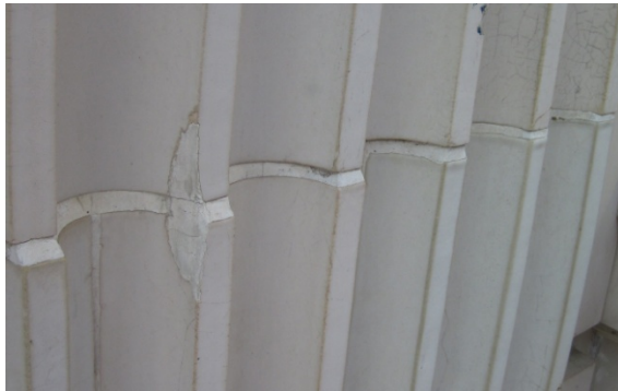
Fig. 25. Showing repointing of joints with hard and impervious polyester resin, a material often observed for filling patches in the terracotta as well.
