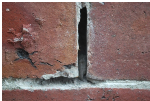
Fig. 11. Behind the recent front pointing which is shallow placed, we see the original mortar is remains voided and will require better repointing supervision next time.
