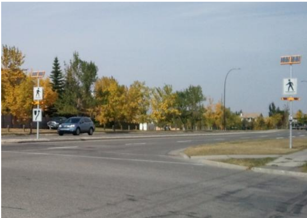
Crosswalk Upgraded with RRFB in Calgary
