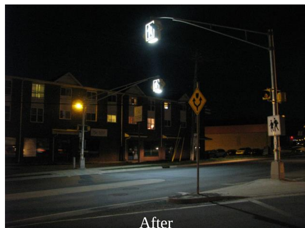
RA-5 Crosswalk on Cole Harbour Road at Bissett Road – Before and After Lighting and Signage Upgrades
