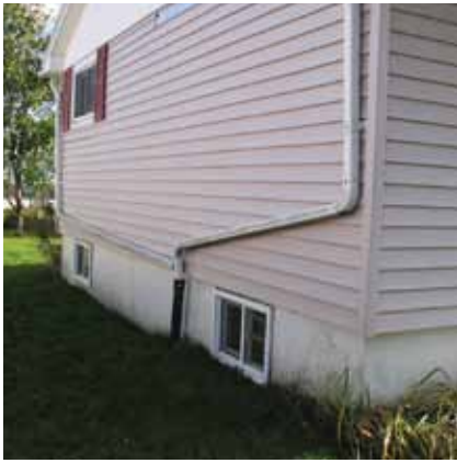
Improper downspout connection
