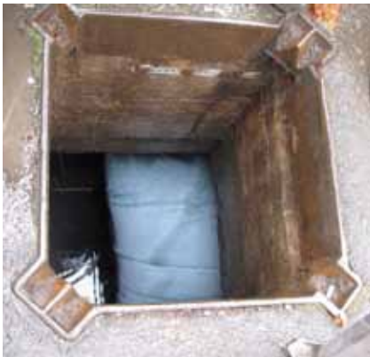
Trenchless pipe liner moving through sewer pipe
