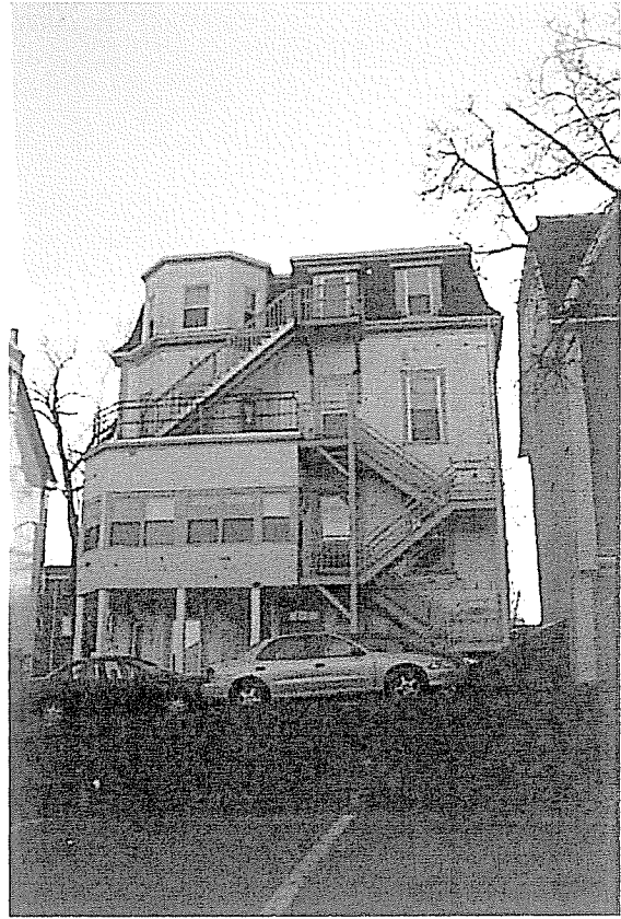
Rear of the Building
