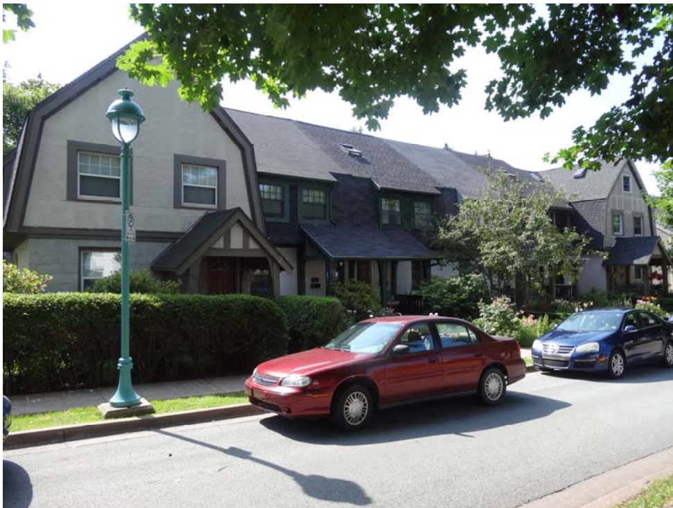
Photo 4 – Typical entry verandas & porticos
