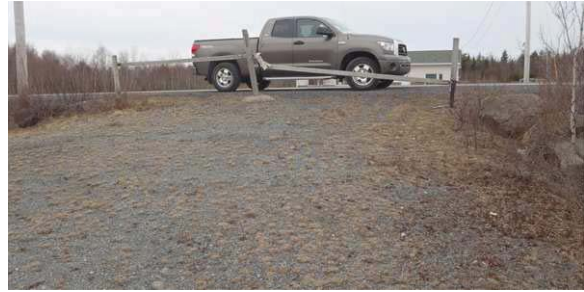
Photo 7: Looking West from Parking Lot toward Driveway 3
